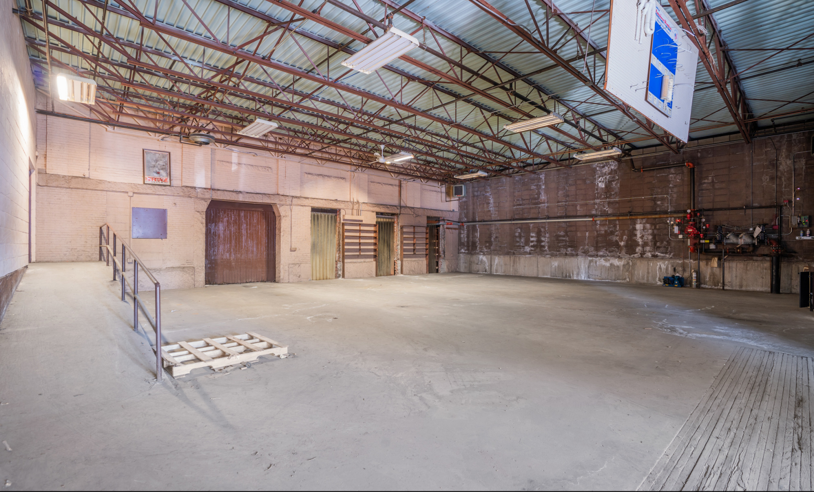
Building 1 - Interior Loading Area
